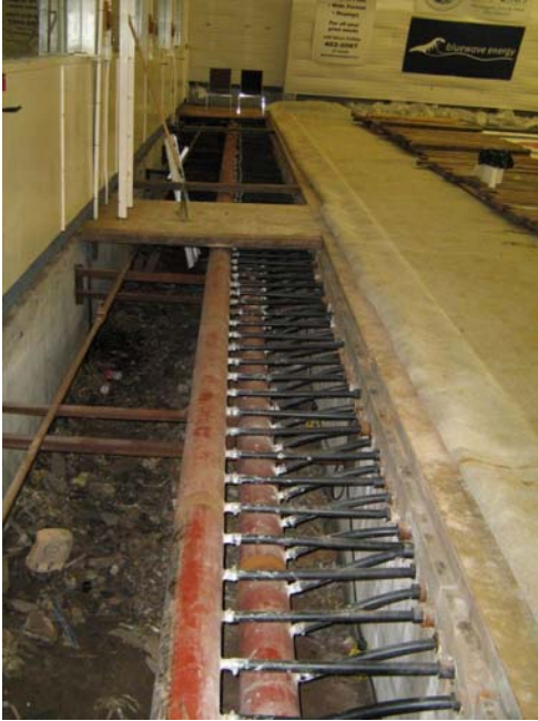
Header pipes Before
